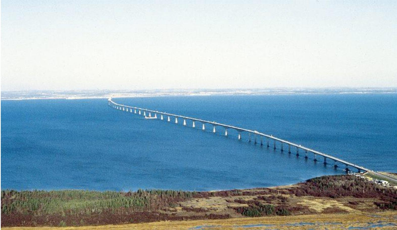
Constructed 1993-97. 0.5 million cubic meters of **special** concrete. 13 km long.
