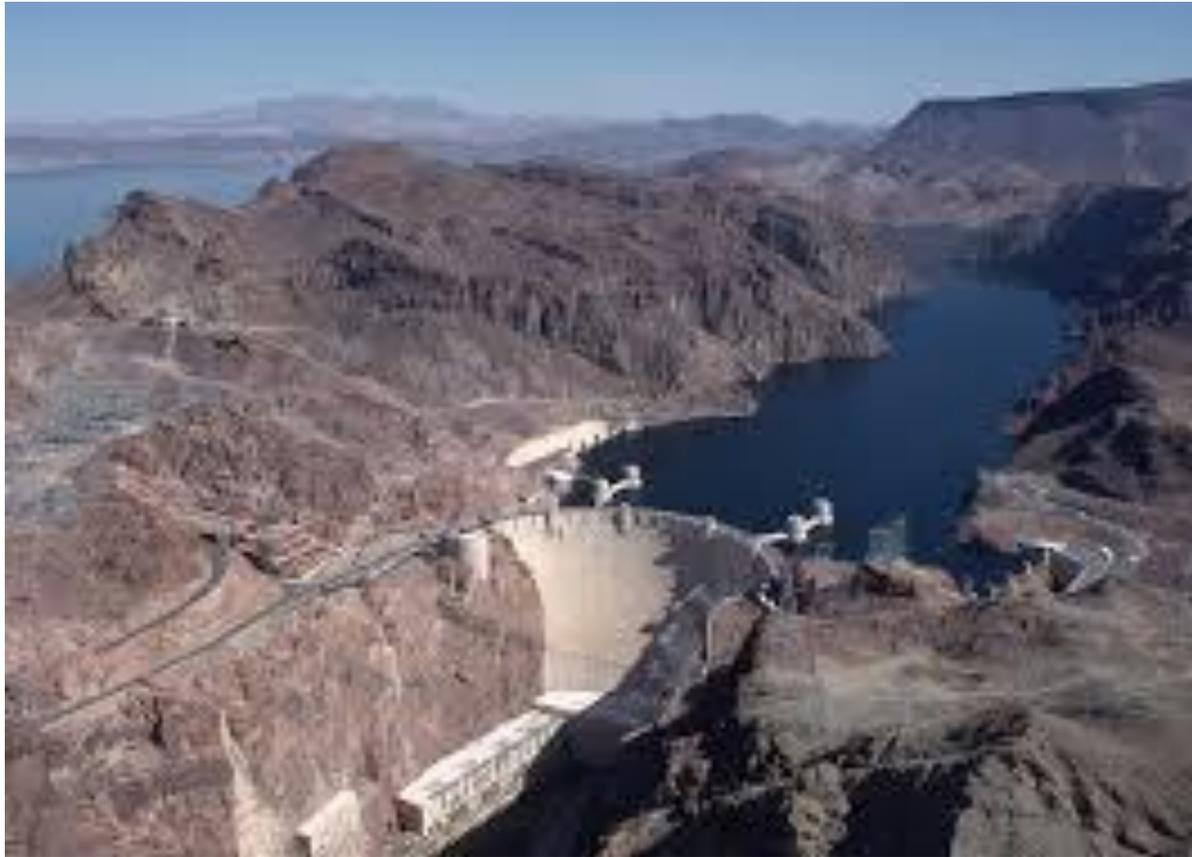
Constructed 1931-36. 2.5 million cubic meters of concrete. 70 stories tall. Provided flood control, water for agriculture, and electricity for southern California, especially Los Angeles. 112 construction workers died in accidents.
