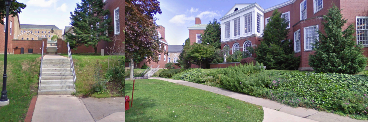
Figure 4: Schwartz Ramp Location (Google Maps, September 2012)
